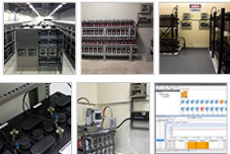
Battery failure can happen overnight, and Eagle Eye's IBwatch-Series real-time battery monitoring allows full protection and confidence against such failures. Ohmic resistance and voltage measurements (per jar) are taken as often as every five minutes. String current, DC voltage, and temperature are measured in real-time. These measured parameters will provide the user a real-time understanding of their batteries state-of-health.
