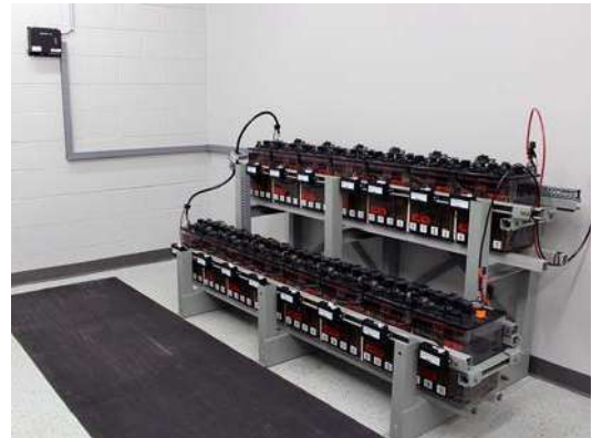
BQMS Installation to 120VDC Battery System
