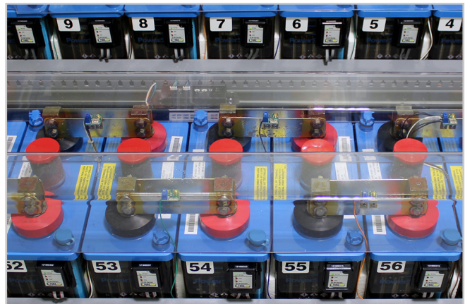
Installation to Battery Cells
